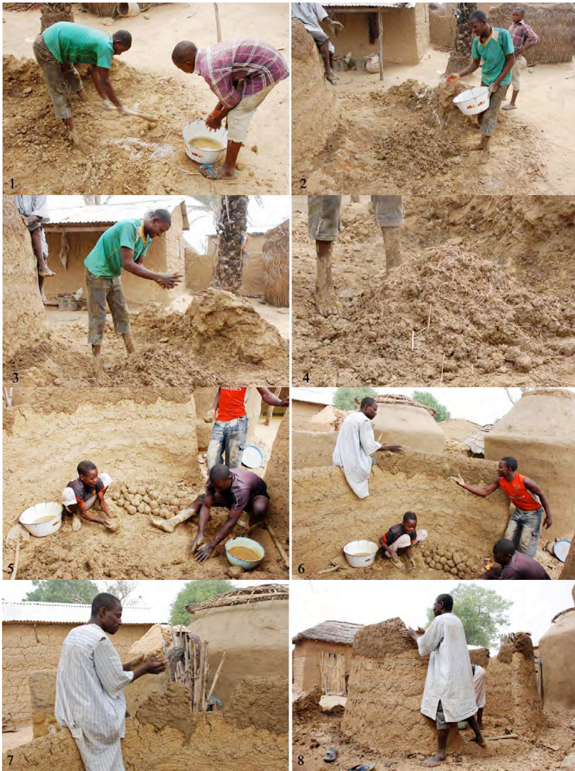
1. Grinding 5. Preparing the bricks by compacting the mixture 2. Watering 6, 7, 8. Building 3. Mixing the earth with straw 4. Making the mixture homogenous
